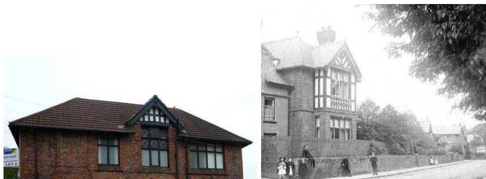
No 52 Bromborough Village Road: The north elevation (left) illustrates the loss of the east and west projecting gables and chimney shown in a 1920s photograph (right). (Note the open space beyond the building is the site of 36-46 Bromborough Village Road)
