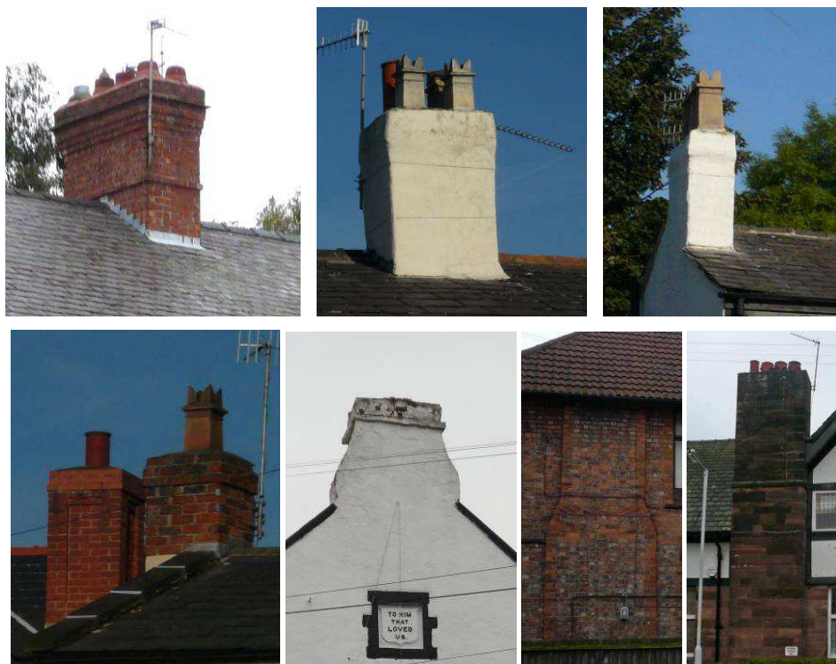
Examples of different chimney types within the conservation area
