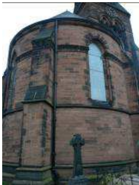
Typical 'Early English' details: paired lancets beneath a large rose window (top left); blind arcading (top right); a buttress to the apsidal east end (bottom left); and a typical window with paired lancets, cusped plate tracery and clustered shafts (bottom right)
