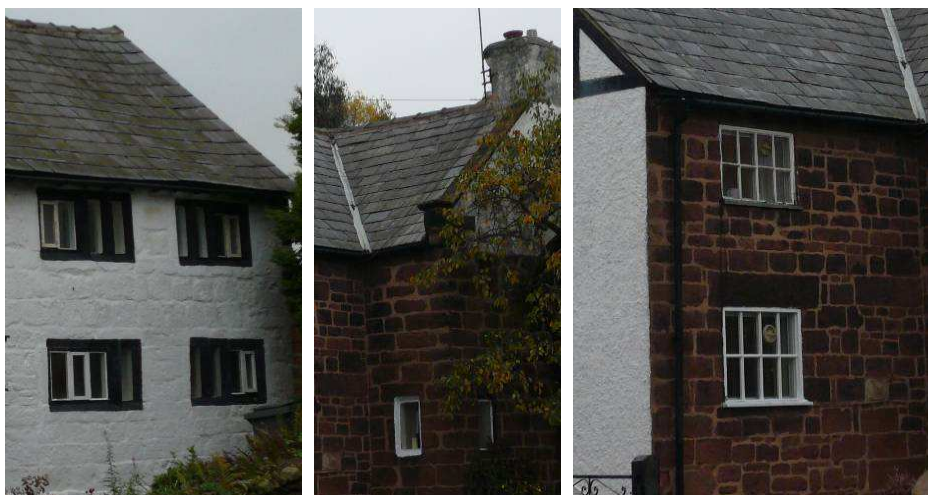
No 6 The Rake (listed grade II):- (left) to the east elevation of the original cottage are 4-light single chamfered mullioned windows (extended at some point), those to the west are single-lights (centre). The windows to the extension are later, being 8-light fixed windows (right). The upper window is probably contemporary with the extension but the lower window is a later replacement.
