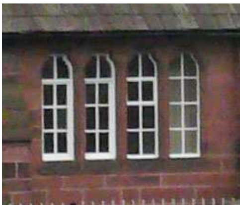
Village Centre windows have lancet openings with shouldered lintels, chamfered sandstone mullions with 8-light windows, and are arranged in groups of two, three or four.
