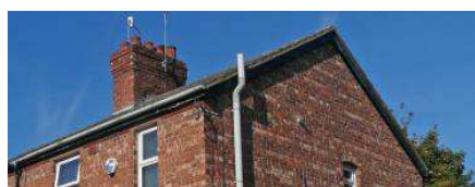
Roof details of dwellings along The Rake: earlier buildings (above) have stone coping to flush verges; later buildings (left) have overhanging verges and projecting purlins
