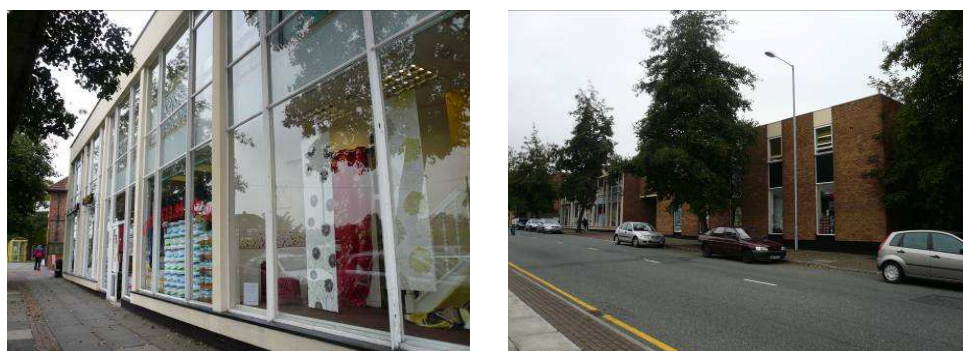
Nos 36-46 Bromborough Village Road viewed from north east: the southern section (left) has a largely glass frontage and the northern section (right) is predominantly of brick
