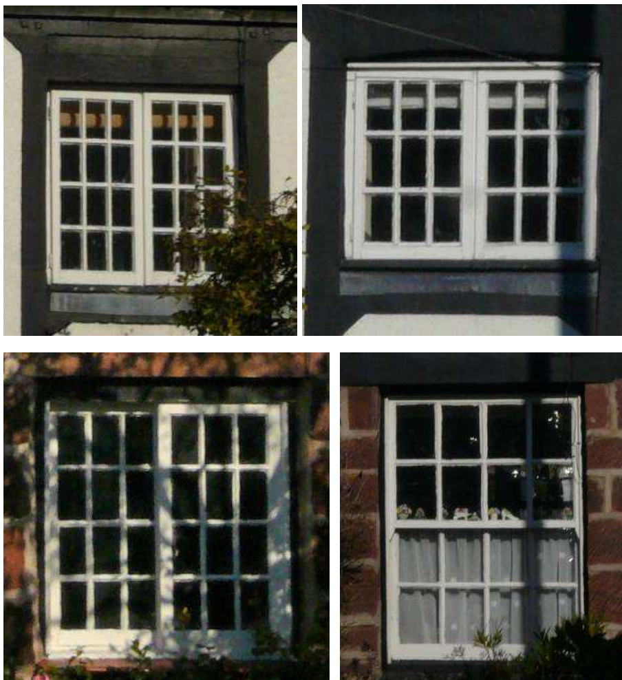
(top left) modern wooden-framed 12-pane casements in square opening; (top right) modern wooden-framed 9-pane casements; (bottom left) a Yorkshire (horizontal sliding) sash in a square opening; (bottom right) 16-pane double hung sash with horns, in an altered opening (possibly the original doorway and contemporary with the later C19th extension to the left)
