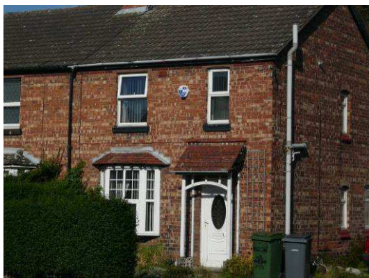
Larger, vertical openings at Nos 2, 4, 12 and 14 The Rake with canted bay windows on corbels to the ground floor, typical of the late C19th/early C20th. The original windows would have been two pane double-hung sashes with horns, though regrettably none remain.
