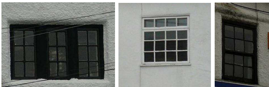
(left) Nos 54-56 Bromborough Village Road, C17th window to dormer; (centre) No 26, square mid-C18th window opening with modern toplight; (right) Nos 54-56, C19th 12-pane double hung sash
