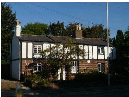
Nos 16 and 18 have been much altered and extended over their lifetimes, illustrated by the unusual variety of window types and openings (see examples below). Although each window is different, they are of an historic form and enhance the character of the cottage.
