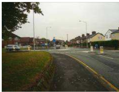
View looking west along The Rake near its junction with Allport Lane (western end)
