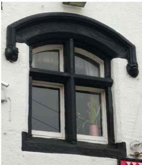
The distinctive 19 th -century Gothic revival windows at 18 Bromborough Village Road have heavy, painted stone, chamfered mullions and transoms with a shallow arched head and carved finials to heavy hood moulds, set with wooden-framed lights.
