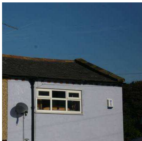
More considered placement of the rainwater downpipe, satellite dish and burglar alarm would improve the aesthetic appeal of this cottage
