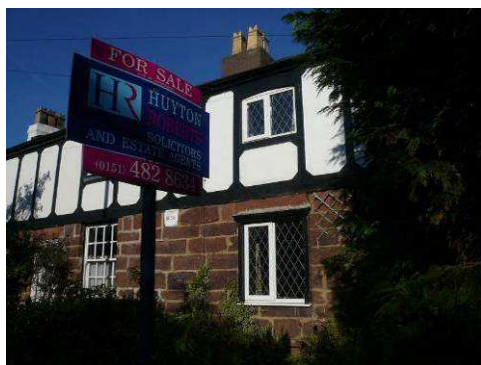
No 16 The Rake: Replacement uPVC two-light windows with single side-hung casements and imitation diamond-shaped leading. The upper window is almost flush with the wall face, instead of being recessed in the same way as the earlier windows to No 18 adjoining. The inserted timber reveal to the lower window stands proud of the wall face and is totally out of context.
