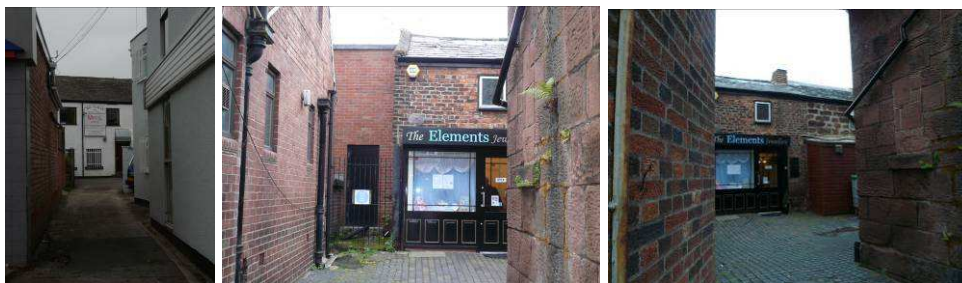
These buildings behind the NatWest bank and former Royal Oak public house may be remnants of the agricultural properties that stood on this site
