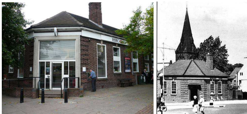
58 Bromborough Village Road: unsympathetic alterations are illustrated by comparison with a photograph from the 1950s
