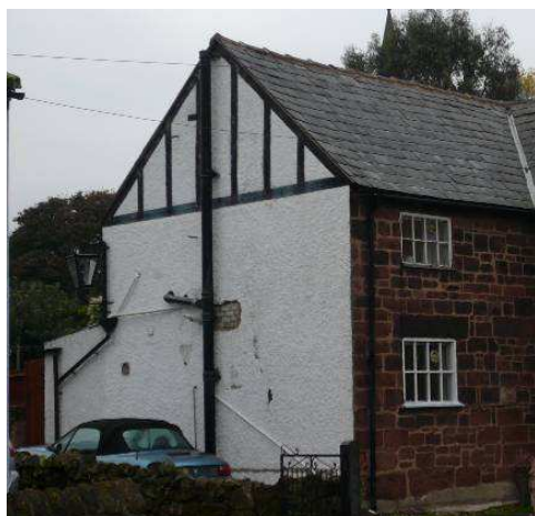
Intrusive waste pipes and rainwater goods
