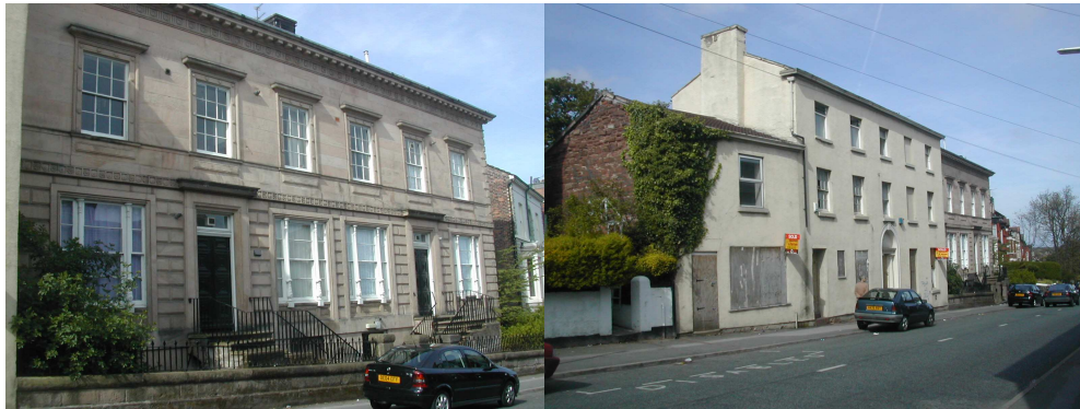
Numbers 140/142 and 144 Whetstone Lane. Although of a similar date and both listed, they are of stark contrast in terms of condition.
