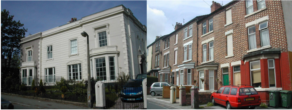
(Left) Grade II listed 34 & 36 Clifton Road. Although generally in a good state of repair, the symmetry of the pair is partly lost due to the unmatching render types and the insertion of top UPVC casement windows into the openings of the left hand house. (Right) Terrace on Brookland Road. The attractiveness of the polychromatic brick is marred by the muddle of different windows, painted brick and cars parked in gardens.
