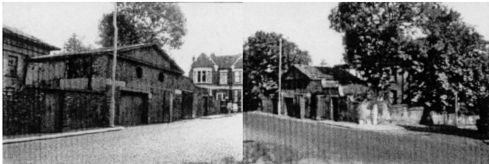
Photographs of coach house on Whetstone Lane, prior to demolition.
