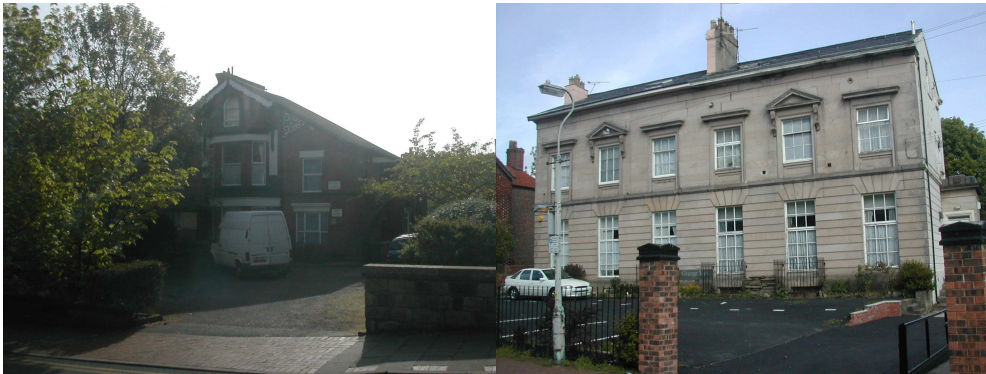
Number 45 Clifton Road (left) and 53 / 55 Woodlands (right). Both examples of larger properties being subdivided into flats. 45 Clifton Road is dominated by parking in front of the building, ugly signage and an external fire escape. 53 / 55 Woodlands has a tarmac parking area taking up virtually all the front area. Its stonework is dotted with extract vents and its roof littered with television aerials.
