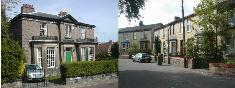
Villa c. 1850 (number 8 Lowwood Grove) and terrace on Circular Road (c.1890)
