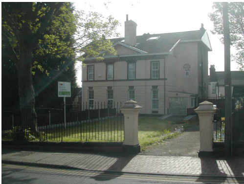
No. 31 & 33 Clifton Road. Although small in scale, an unsympathetic porch with large patio doors is stylistically out of keeping with the rest of the building and upsets the symmetry of the building as a whole.
