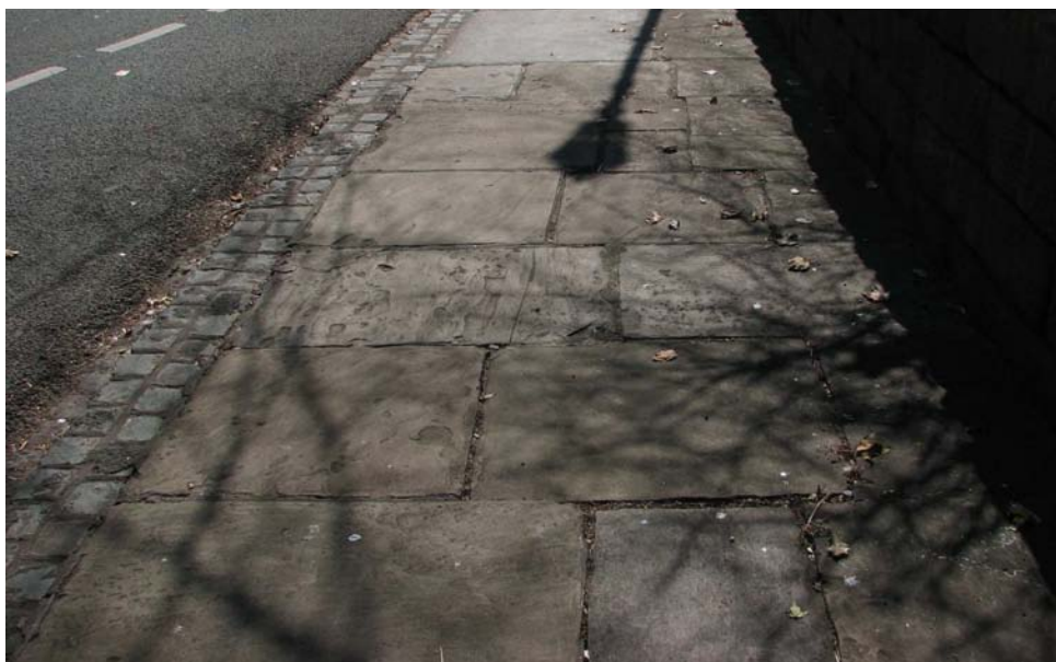
Paving on the corner of Eastham Village Road and Church Lane
