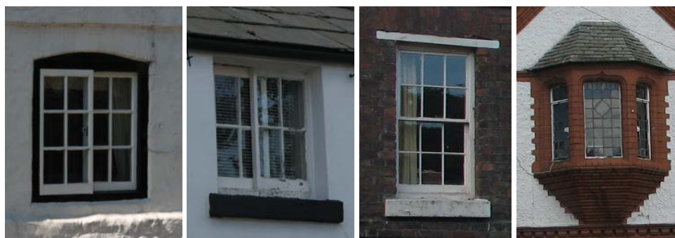
Windows within the conservation area. (1) and (2) show horizontal sliding sash windows, (3) vertical sliding sash windows and (4) leaded windows to the vicarage.
