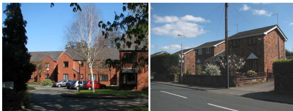
(left) Eastham Mews housing; (right) Vicarage Row
