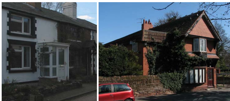
(left) the additional of a porch onto the front of a terrace can be damaging to the visual rhythm in the group; (right) a larger extension which changes the character of a building.
