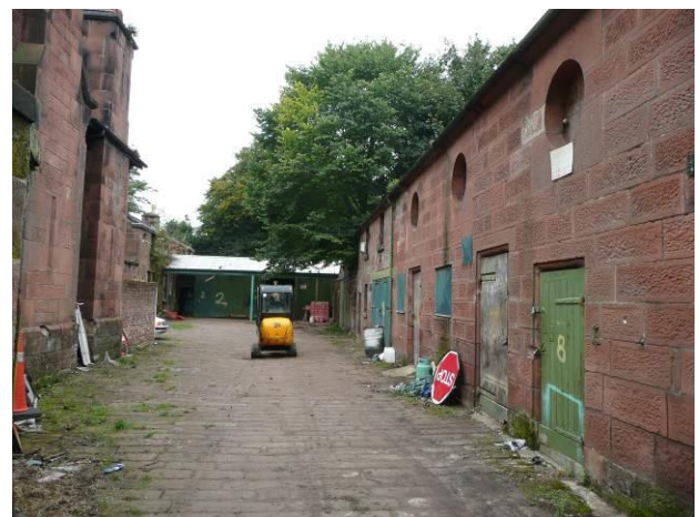
Old barn storage
