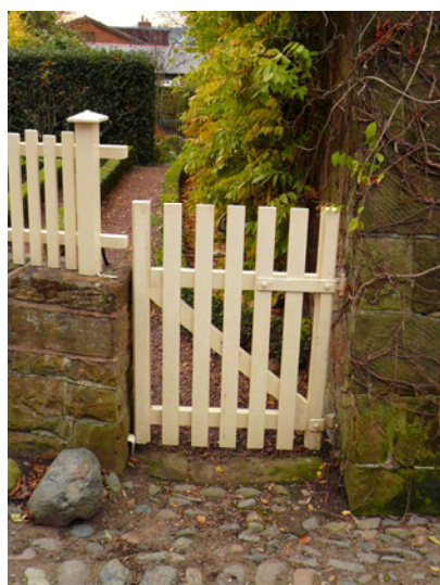
Roughly coursed sandstone walls, a simple picket fence and a gate inserted into a wall with no gate posts are all appropriate to the modest vernacular context. The wall on the right is in a poor state of repair and has been badly pointed.
