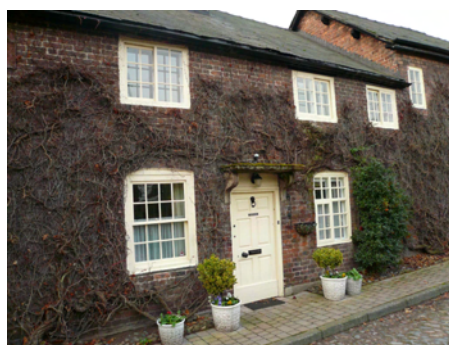
Vertical and horizontal sliding sash windows and casements can all be seen on one building here at The Old Farm. The window openings are unadorned.
