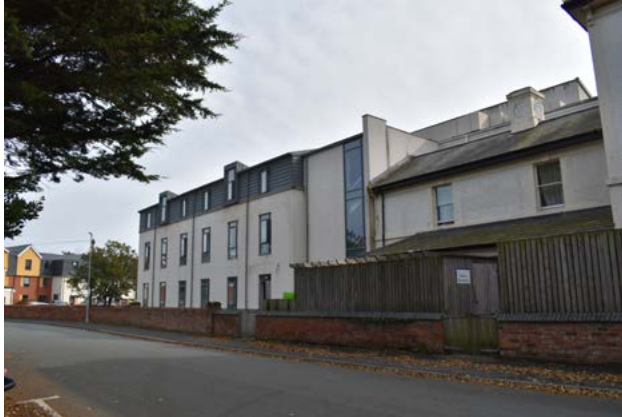
6.5 Poor quality extensions and new buildings replacing historic fabric and eroding inherited street patterns
