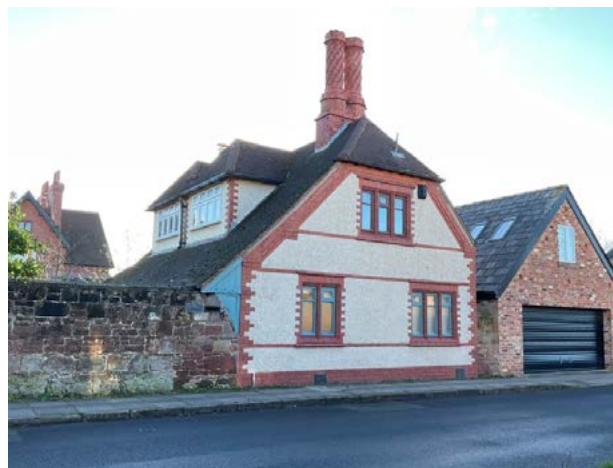
4.4.24 Former coach house to the rear of 32 Stanley Road
