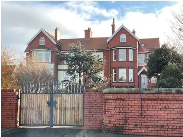
4.6.5 Red brick building with white rendering to facade
