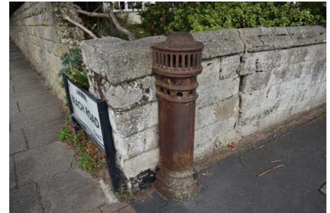
4.4.28 Victorian stink pipe to the junction of Beach and Stanley Roads
