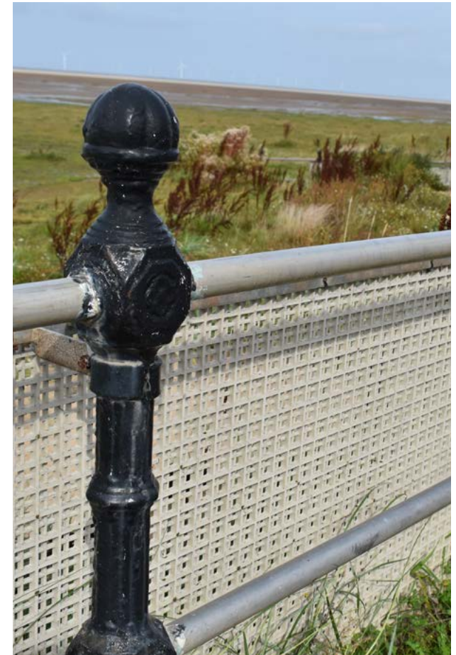
4.6.12 Promenade cast iron decorative railings
