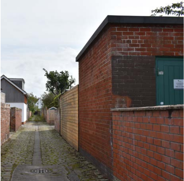
4.7.12 Detrimental substation off Valentia Road
