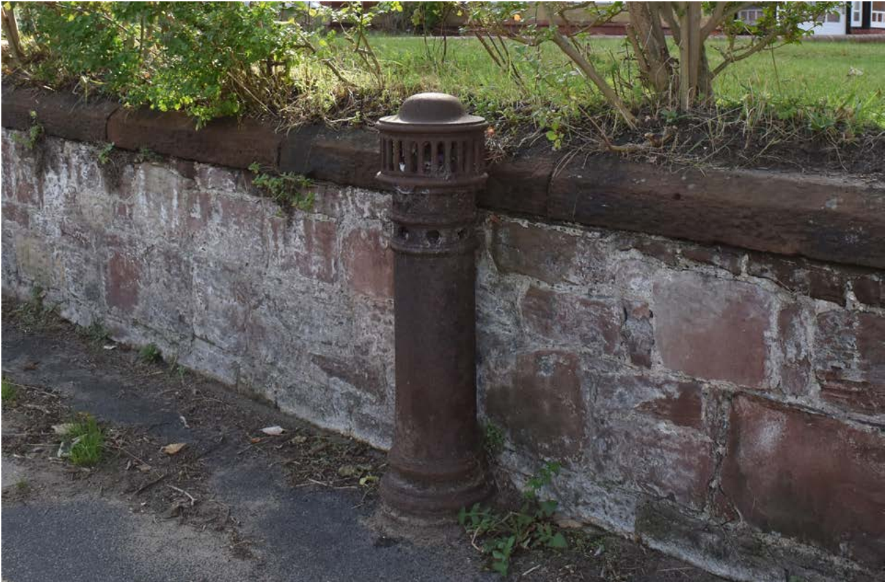
4.5.18 Surviving Victorian sewage pipe on King's Gap
