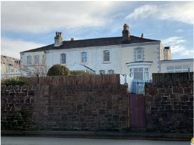
4.6.7 Quoin detailing on North Parade
