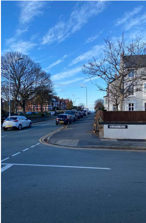
4.3.22 Views north to the coast from the junction along The King's Gap
