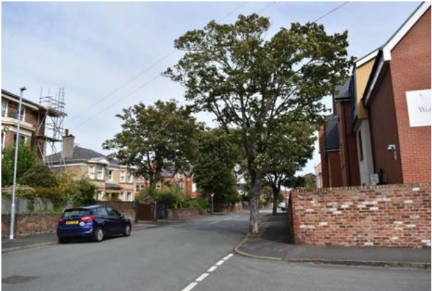
6.3 The scale, massing and poor quality of Westhaven Care Home disrupts the aesthetic and historic street pattern
