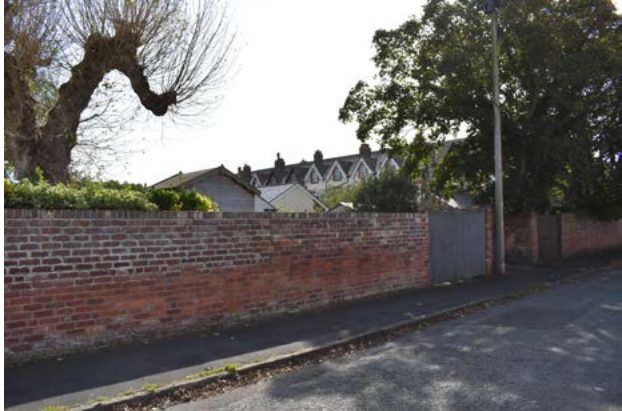
4.7.11 Marine Drive high brick boundary wall
