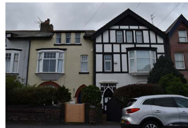
6.1 Loss of detailing to windows and the rendering of the terrace on Alderley Road reduces its legibility
