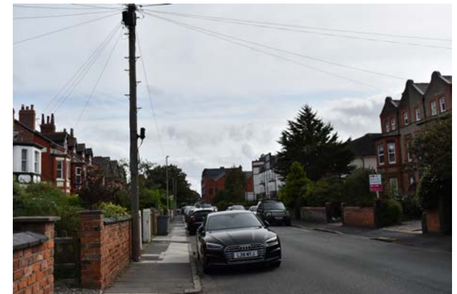
4.7.18 Southwest view along Queen's Road towards Town Hall
