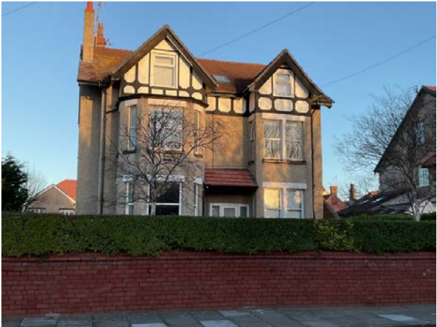
4.5.11 Timber studwork on Curzon Road building
