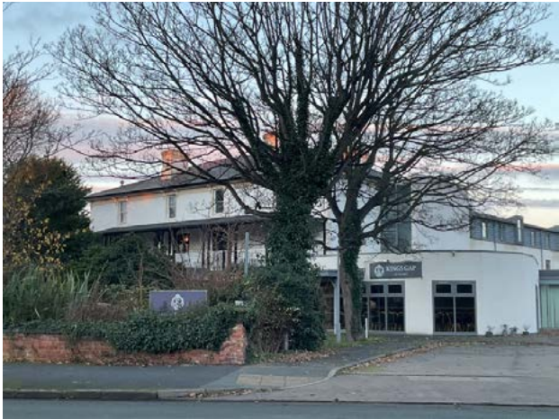
4.3.6 Former hotel, The King's Gap
