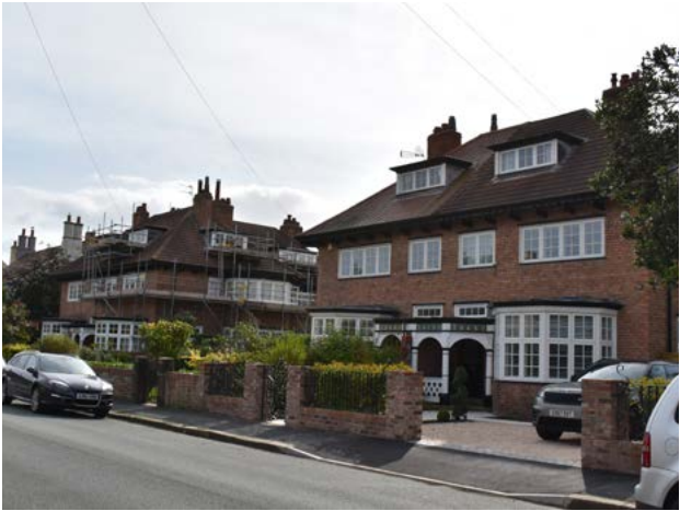
4.7.9 25-27 and 29-31 Cable Street
