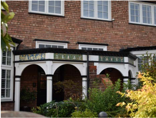
4.7.10 Tiled detailing to 25, 27, 29 and 31 Cable Street
