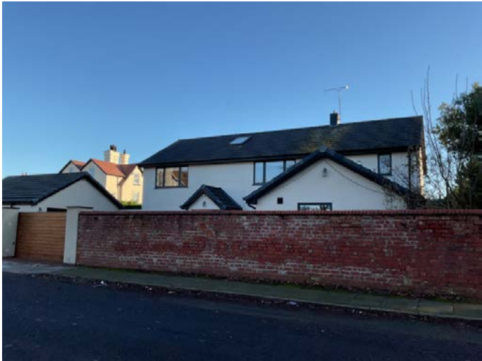
4.4.27 33 Barton Road, modern dwelling
