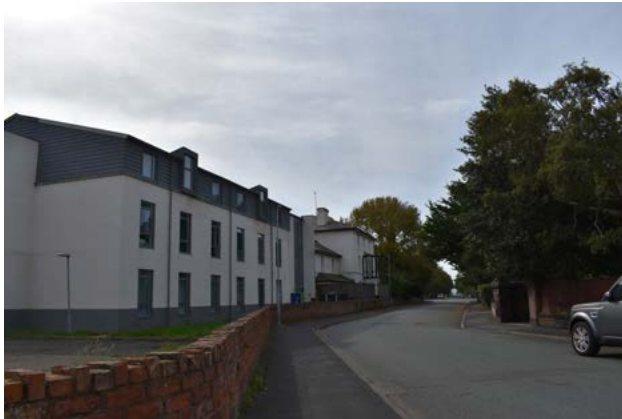
6.2 Higher level building at The Holiday Inn
