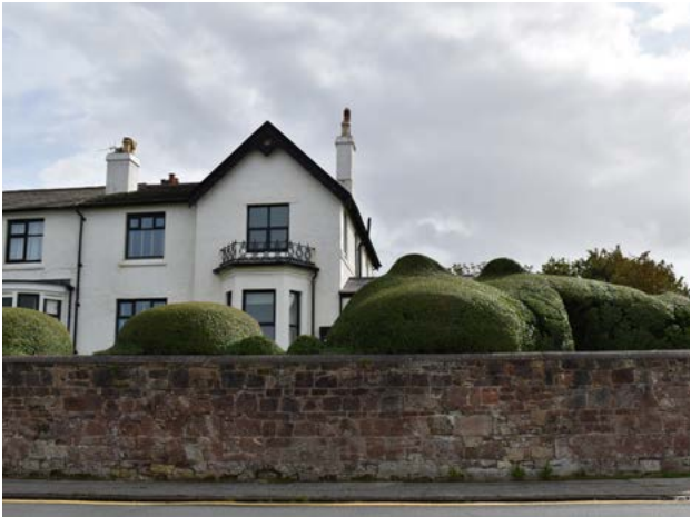
4.6.4 North Parade typical building
