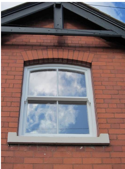
New sash window, again in Bromborough Pool. Note later details such as larger panes and horns to strengthen the connection with the mid-rail now that only one vertical glazing bar is present to secure it.
