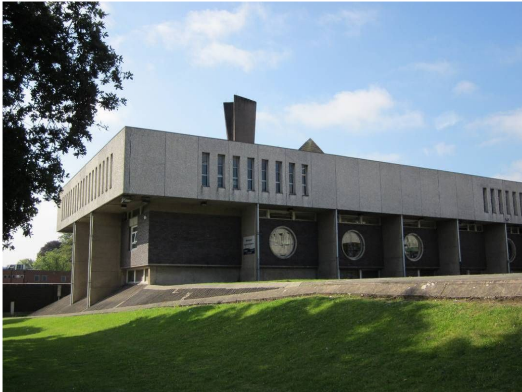
The Civic Centre – showing library, with upper floor on podium and porthole windows to ground floor; funnel boiler chimney and pyramidal roof to atrium.
