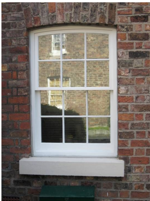
New double-glazed timber sash window, installed in Bromborough Pool Village as part of comprehensive upgrading by Riverside Housing. Beauty and efficiency effortlessly combined – note wavy handmade glass on exterior of d-g units, giving increased privacy and optical character.
