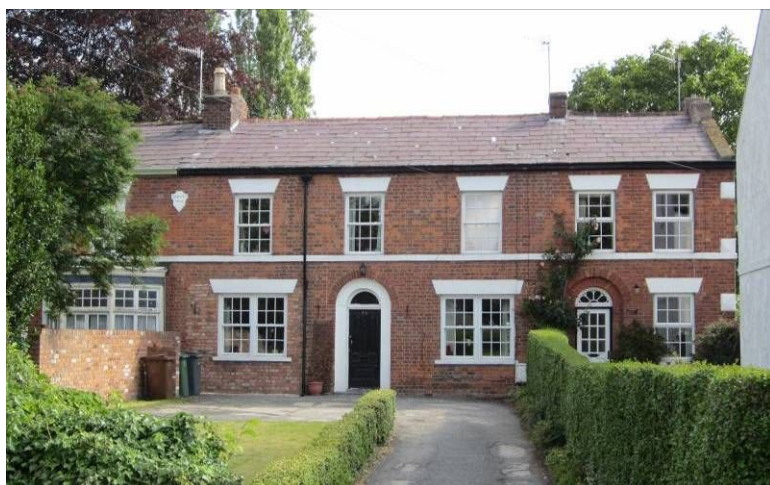
Park View Terrace – fairly standard yet refined early Victorian terrace. The paired sash windows to the ground floor are relatively unusual for the time; dated 1852.
