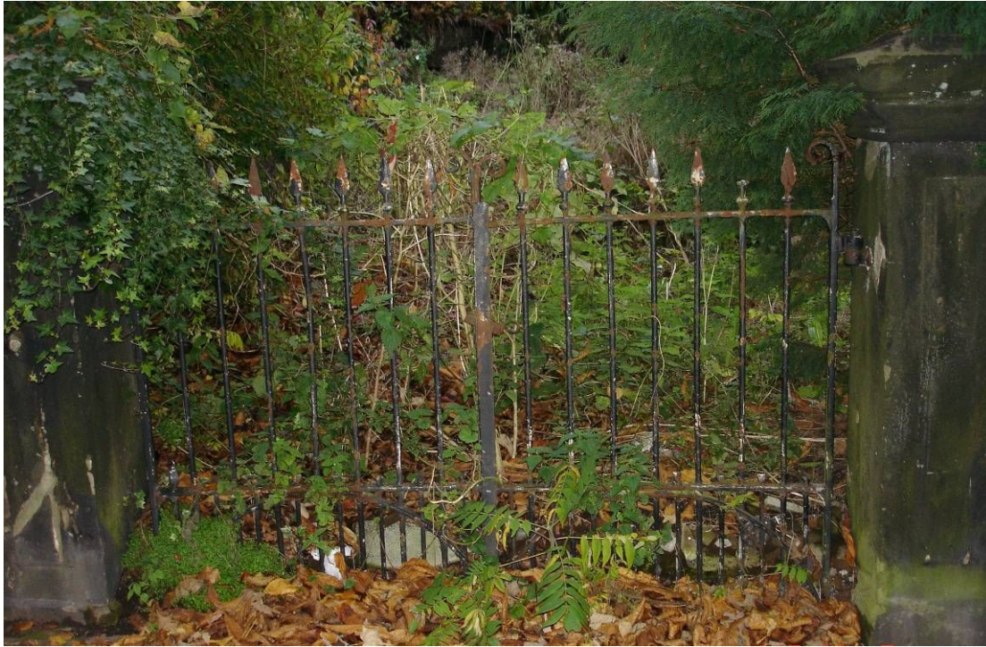
Traditional iron gates and sandstone gateposts to The Grange, Acres Road
