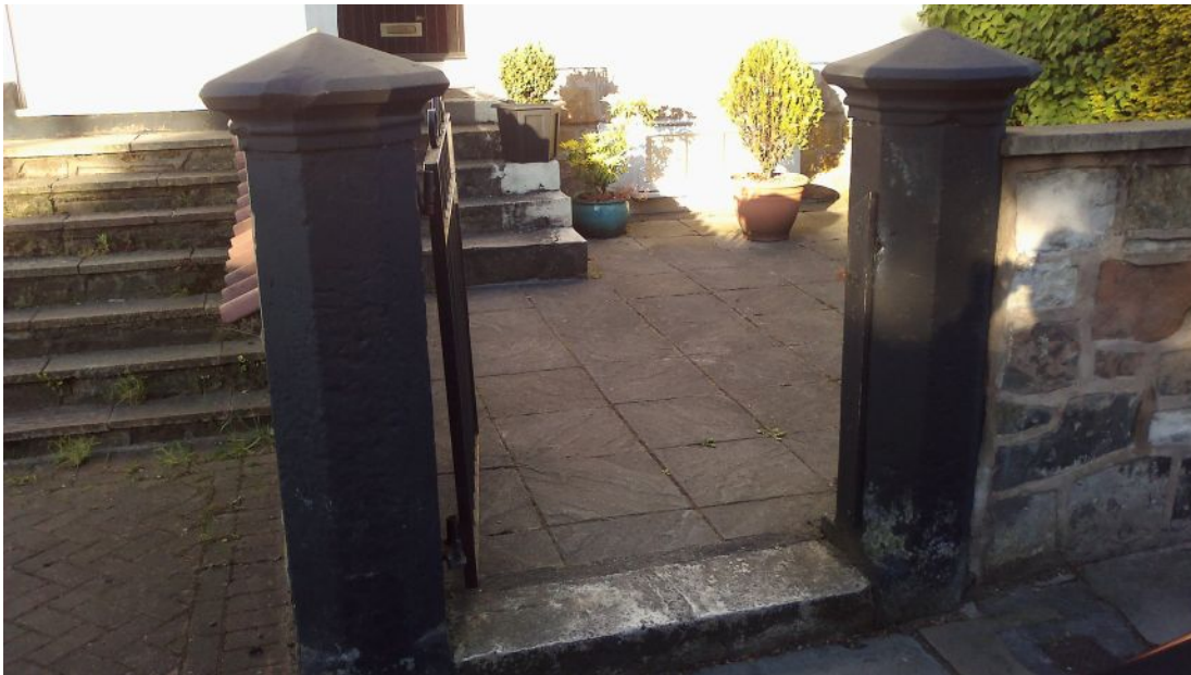
Typical Regency carved stone gateposts, Mersey Terrace.
