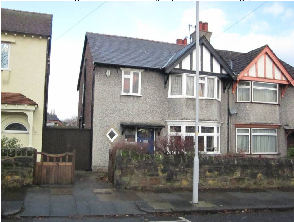
Stone rubble front boundary wall, with triangular stone copings and timber gate. Note gentle upwards curve of wall towards entrances.
