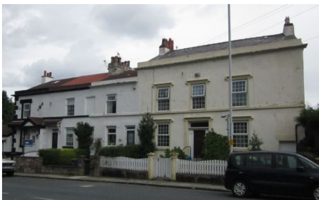
Mersey Terrace – neoclassical Regency terrace in lime stucco render, with: end-gable chimneys, slate roof, parapet gutter and cornice with blocking course above (to support heavy cornice), hood moulds over windows, sill band to 1 st floor windows, some evidence of architraves, low stone wall and stone gate piers, fanlight over door and panelled pilasters either side of front door (sadly replaced).
