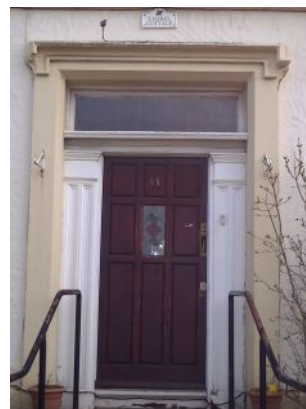
Mersey Terrace – neoclassical Regency terrace in lime stucco render, with: end-gable chimneys, slate roof, parapet gutter and cornice with blocking course above (to support heavy cornice), hood moulds over windows, sill band to 1 st floor windows, some evidence of architraves, low stone wall and stone gate piers, fanlight over door and panelled pilasters either side of front door (sadly replaced).
