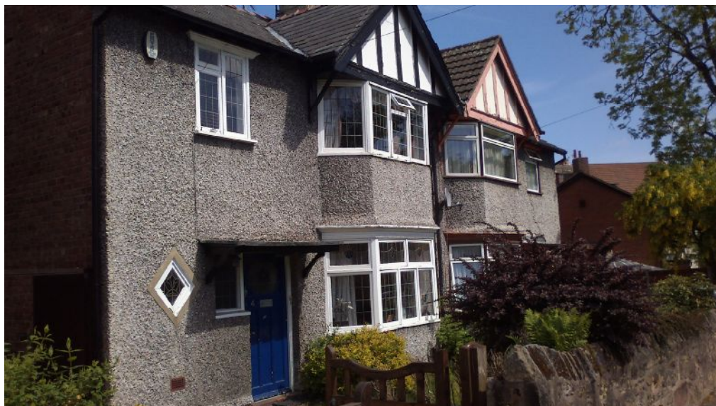
Note the contrast in appearance between the original flush-fitting inter-war timber windows on the l-hand property and the unsuitable later replacements on the r-hand property. The horizontal character of the latter is totally out of place.
