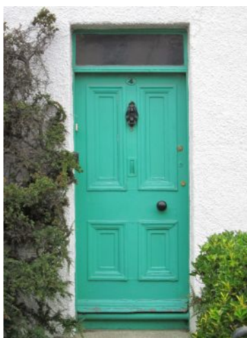
Simple but similarly original four panelled mid-Victorian door. Note inserted letter box, installed when national deliveries were introduced. Fine joinery let down by synthetic green paint colour.
