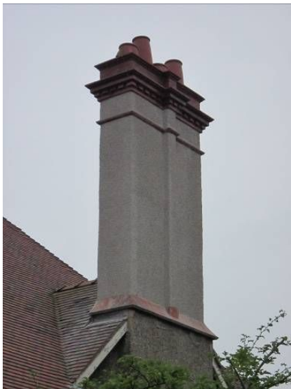
Tall chimney with ornate corbelling on one of the manager's houses on The Wiend.
