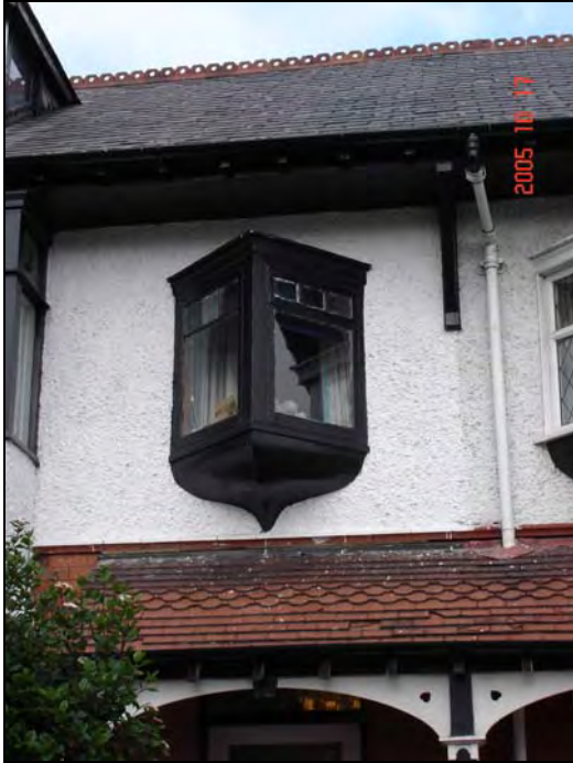
Timber oriel & clay tiles, Vaughan Road
