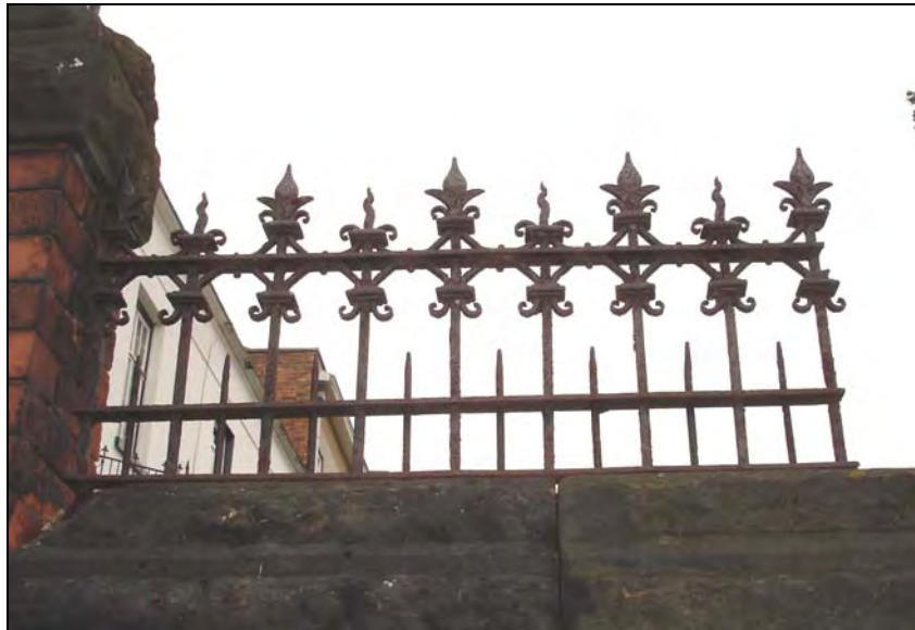
Plate 9 - cast iron railings, no. 1 Marine Terrace
