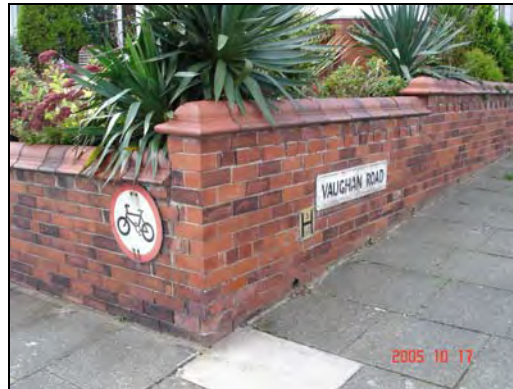
Terracotta coping, Vaughan Road
