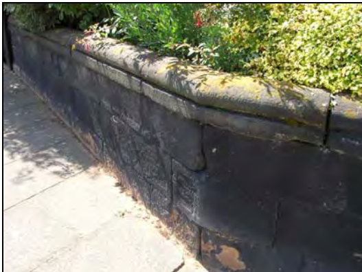
Fine sandstone wall & coping, Magazine Brow
