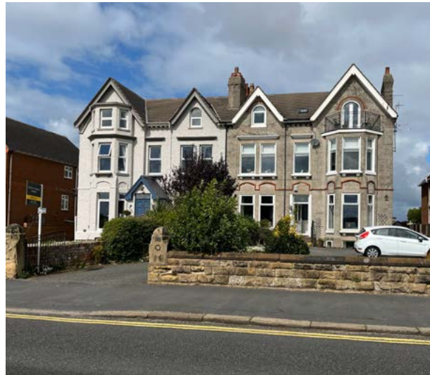
7.4.1 Historic property on Stanley Road
