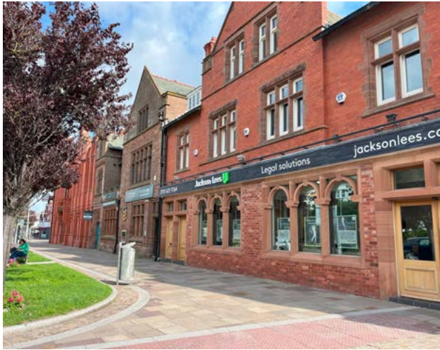
4.4.7 The Quadrant along Market Street
