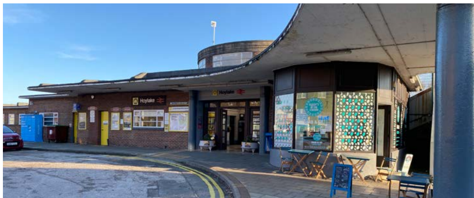
2.1 Hoylake Rail Station
