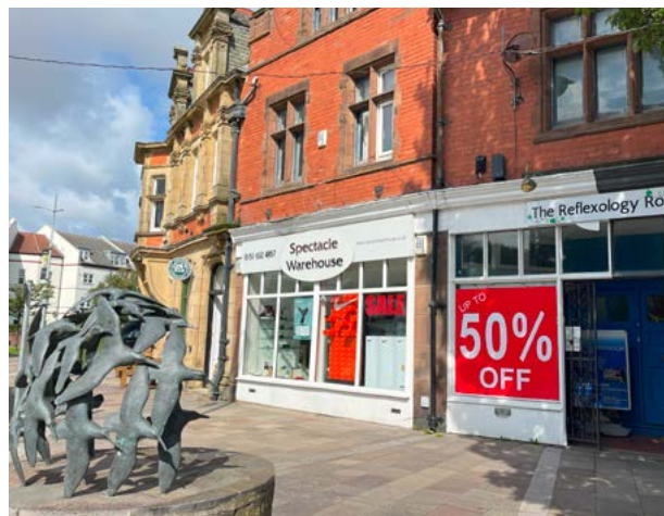
6.8 Key detailing on The Quadrant, including signage encroaching on windows, needs addressing
