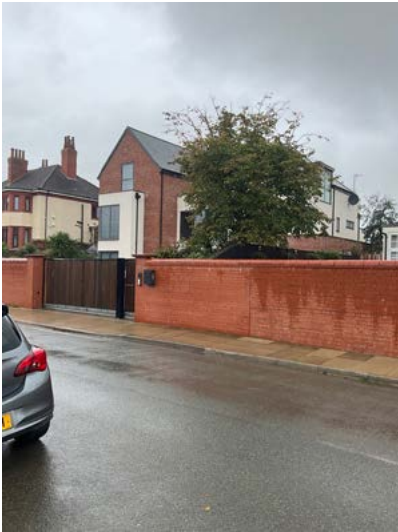
4.3.52 Modern apartment block, Lingdale Road, showing the impact of a high boundary wall and gate
