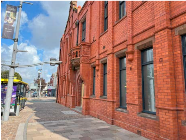
4.4.10 The Town Hall, Market Street
