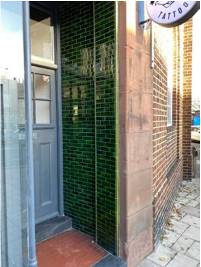
4.4.9 Tile detailing at The Quadrant
