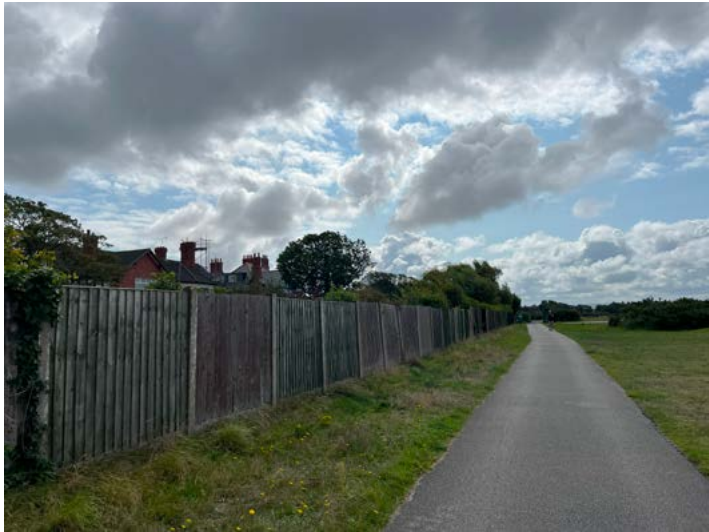
6.5 Poor means of enclosure on key spaces (e.g. golf course)
