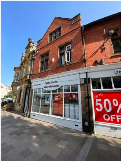
4.4.8 Example of window replacements along The Quadrant
