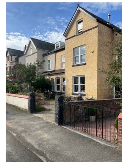
4.3.29 Vertical detailing, Drummond Road
