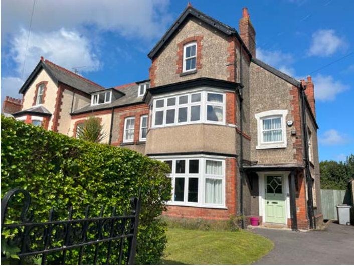
4.3.49 Mixture of brick and roughcast render, with vertical detailing, Lingdale Road
