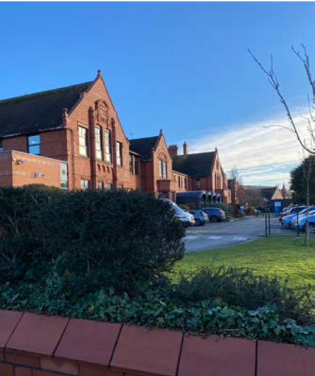
4.5.7 Views to the school frontage are filtered through trees
