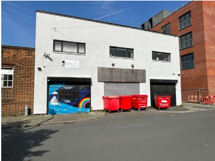
4.4.15 Poor quality building on The Quadrant
