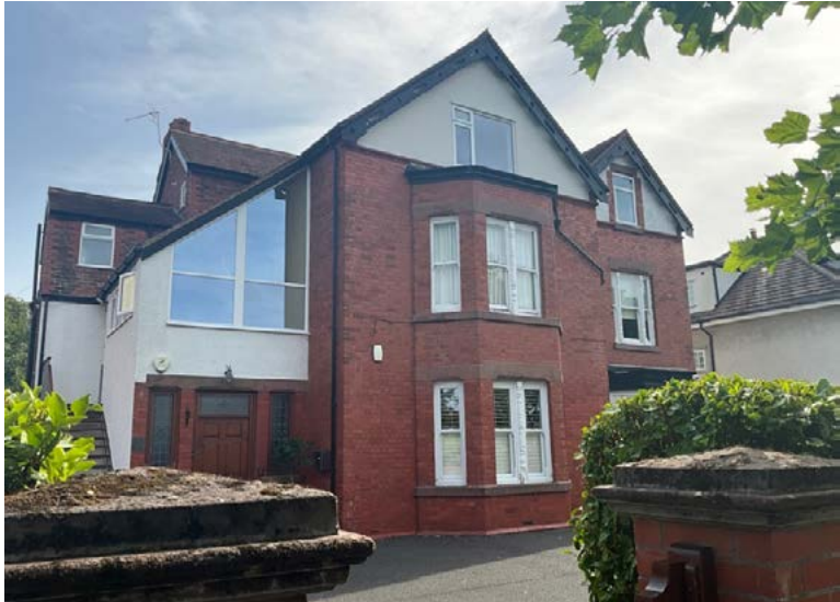
4.3.5 Surviving historic property with substantial later extensions and side escape stairs
