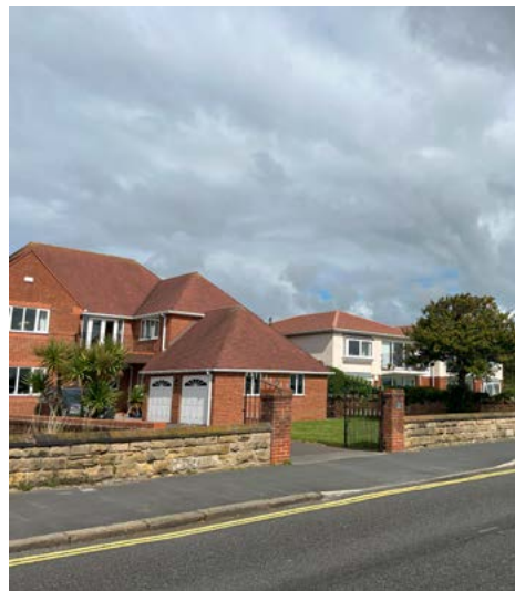
7.4.3 Modern properties on Stanley Road are well scaled and visually prominent from key spaces (e.g. golf course)
