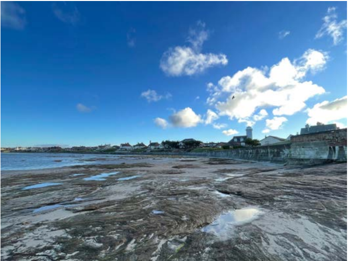
4.6.12 Northern coastline and masonry sea wall
