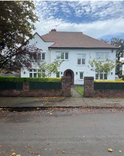
4.3.35 Interwar property with arched door detail, Eddisbury Road
