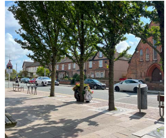
4.4.20 Public Realm works along Market Street
