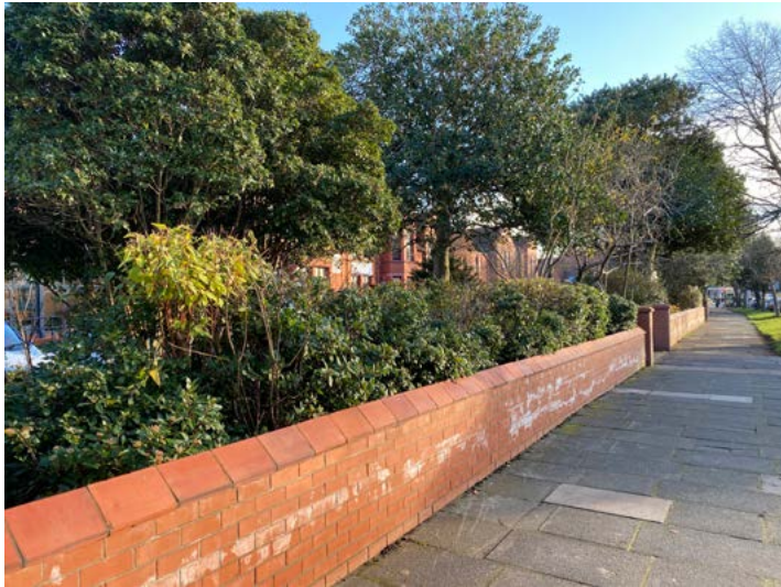
4.5.7 Views to the school frontage are filtered through trees
