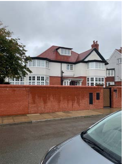
4.3.50 Early 20 th century property, Lingdale Road, with enlarged boundary wall
