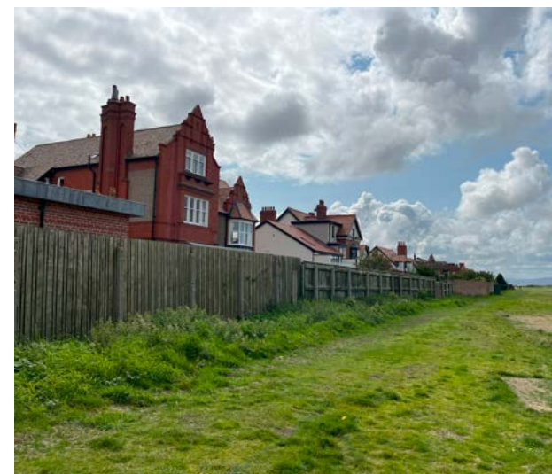
4.7.16 Features such as vertical gables and chimneys are prominent
