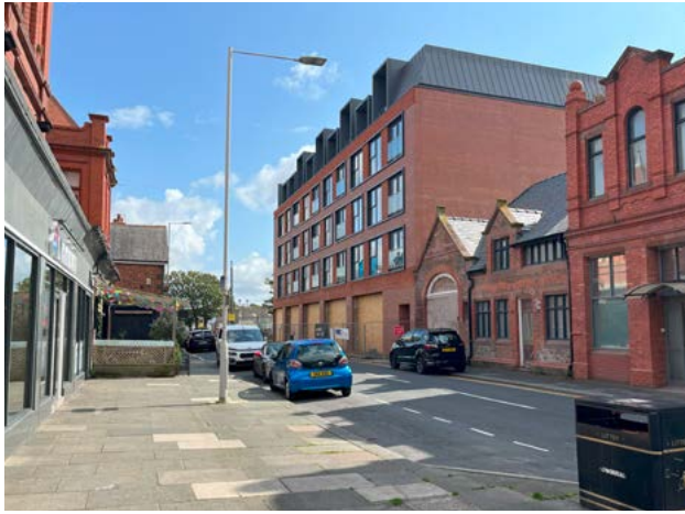
4.4.12 Ongoing redevelopment of the Fire Station site, Fire Engine House also shown (right)
