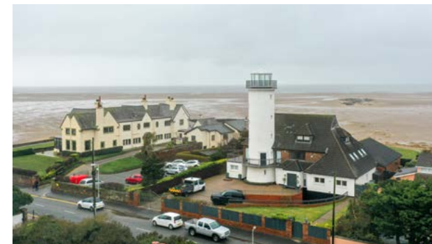
4.6.4 Red Rocks Nursing Home and the modern Hoylake Lighthouse along Stanley Road
