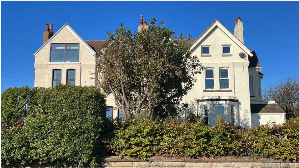
4.6.9 Late 19 th century property, Stanley Road, with altered gables
