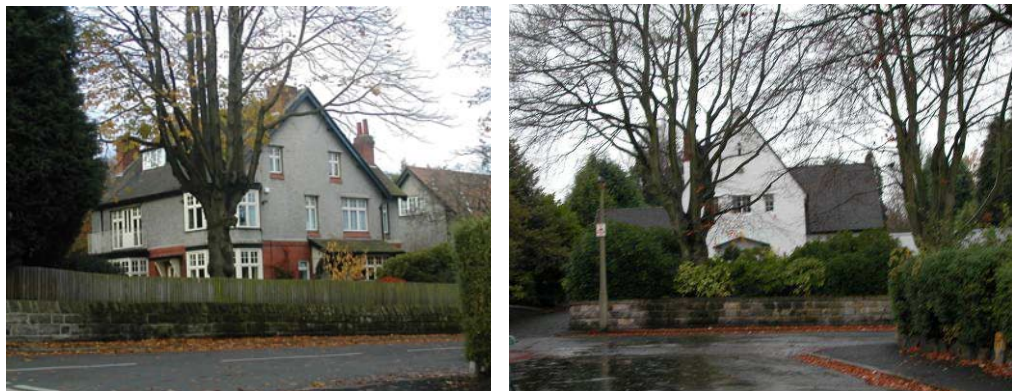
18 Prospect Road as seen from Burrell Road Beech House as seen from Acrefield Road
