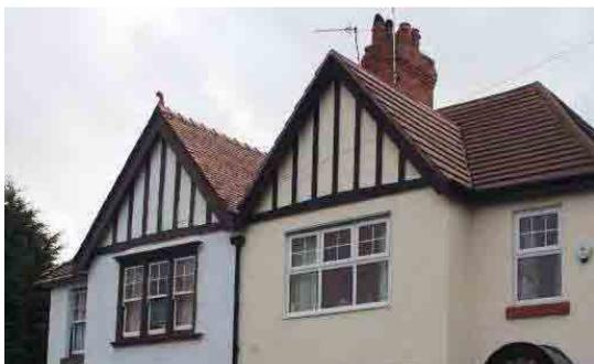
*This pair of houses on Glenmore Road illustrate the impact of replacement windows and roof covering (right) as compared with the originals (left). Concrete tiles have a harsh stepped appearance. The decorative finial and subtle pattern of lapped ridge tiles have been lost. The replacement uPVC windows are flat and lacking in the attractive modelling of sashes with horns, cill and cornice detail and vertical rhythm of sash boxes.*
