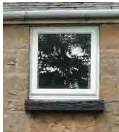
*Early C19th plain small square window opening with sandstone cill set immediately under eaves, with modern window fitted*
