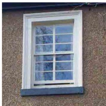
*Double-hung sliding sash window with rectangular panes set horizontally and set back in moulded architrave*
