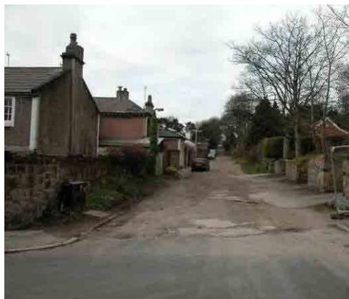
*Arno Road West of Fairview Road is unmade, but heavy use has led to the creation of potholes and some uncoordinated patch repairs*
