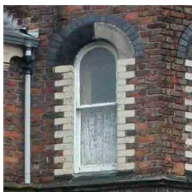
*Two-pane sliding sash with segmental brick and sandstone arched head over projecting sandstone cill band with 'dogtooth' and polychromatic detailing*
