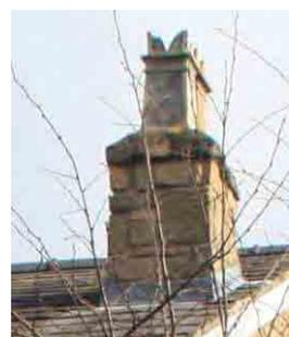
*Small, simply detailed stone-built chimney stacks*
