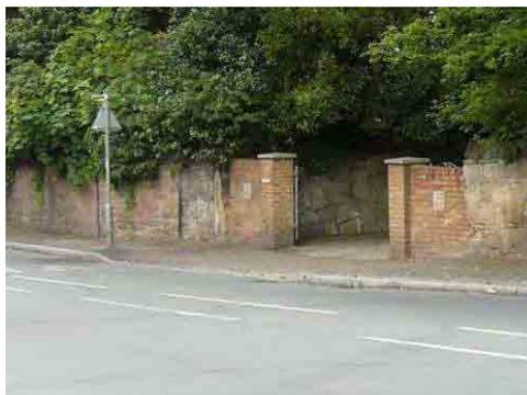
*Inappropriate brick infilling and 'crazy paving' retaining wall behind*
