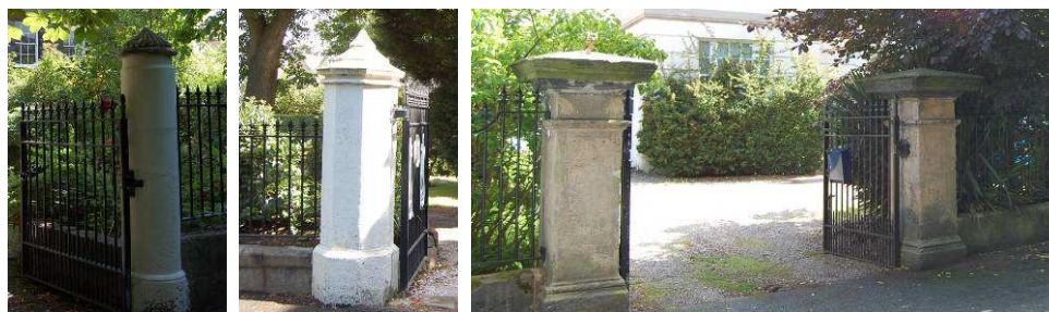
Original gatepost and boundary wall treatments
