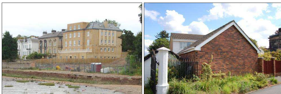
Development in the conservation area which is detrimental to its character or to the setting of its listed buildings: (left) new flats adjacent to 1 Rock Park; (right) Nova House on Rock Park Road
