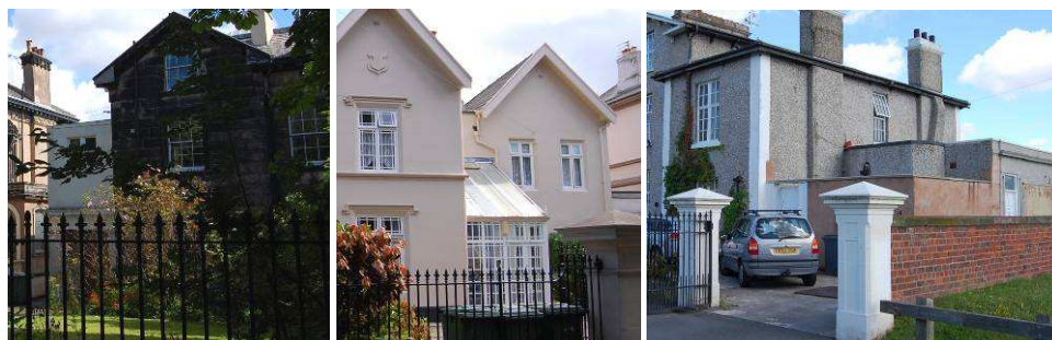
Extensions within the conservation area. The first two images show extensions of a similar form to elements of the original building, but lacking the quality of detailing, the third shows very poor quality and highly visible single storey additions.
