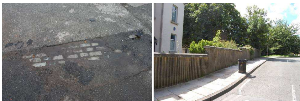
(left) granite setts beneath tarmac; (right) modern concrete slab pavements with concrete walling, presumably constructed at the time of the by-pass
