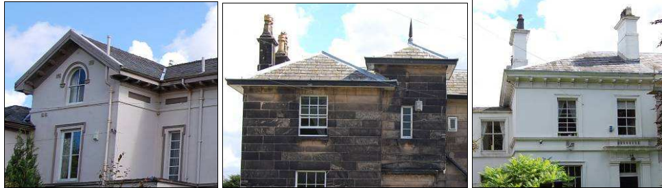
Roof details in the conservation area
