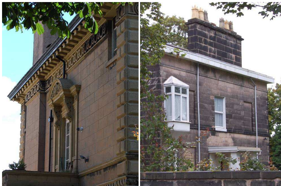
Photographs illustrating the detrimental impact of inserting new openings. The left-hand example shows a small window penetrating through the decorative cornice, the right shows an oriel window (possibly older) and a modern canopy that have unbalanced and changed the architectural quality of the façade. Both of these facades are particularly prominent.
