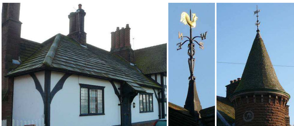
Roof details in the conservation area
