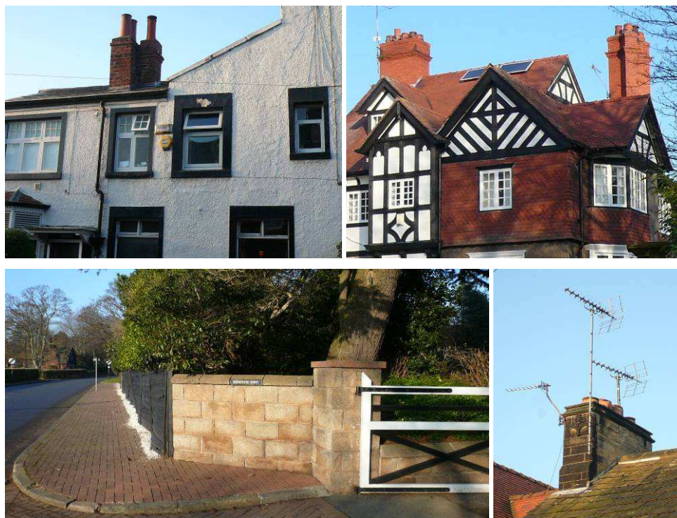
(top left) replacement UPVC windows on the side elevation of the listed Seven Stars public house; (top right) solar panels on the prominent front facing roof slope of Weald House; (bottom left) a modern poor quality fence and wall on Manor Road; (bottom right) large, prominent aerials.
