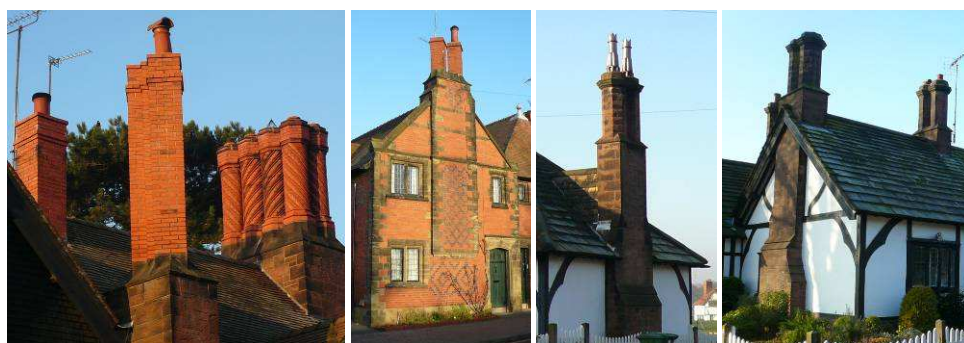
Chimneys within the conservation area.
