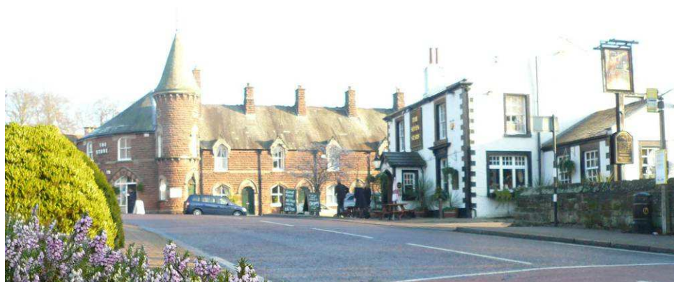
Similar view taken in late 2007 – differences include the loss of the dormer windows on the terrace and the removal of the parapet detail to the public house and the changes to its colour scheme.
