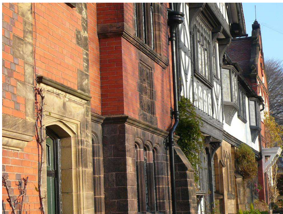
The richness and variety of materials of Thornton Hough illustrated in a single terrace: Buff sandstone, red sandstone, red brick, polychromatic brick, timber framing and pargetted render are all seen here.
